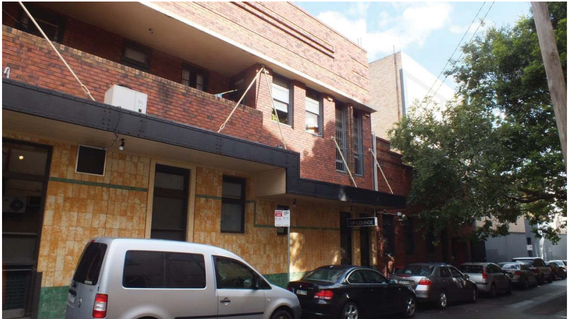
Figure 4 — the north-western elevation, sees from Dunblane Street. Cracks in the brickwork may indicate deflection in the concrete slab. NBRSPARTNERS April 2014
