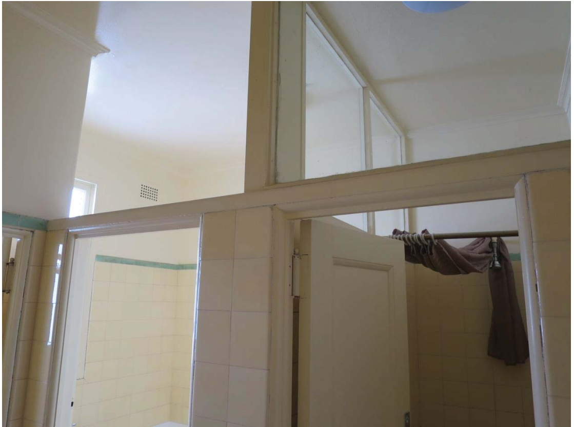
Figure 14 — view inside the women's bathroom showing original tiling and painted joinery.
