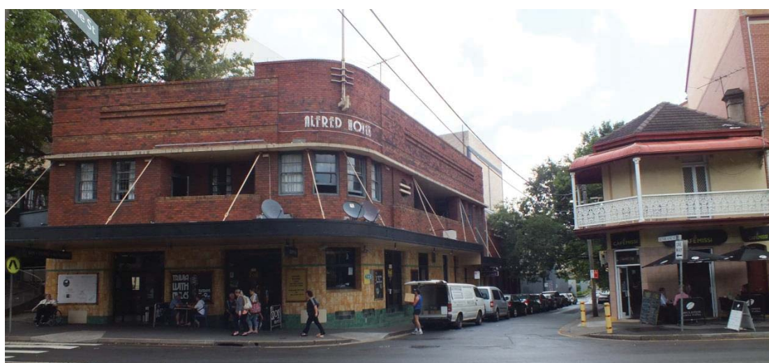
Figure 3 — the subject site on the left, and an altered Victorian shop is on the right, seen here from Missenden Road. NBRSPARTNERS April 2014
